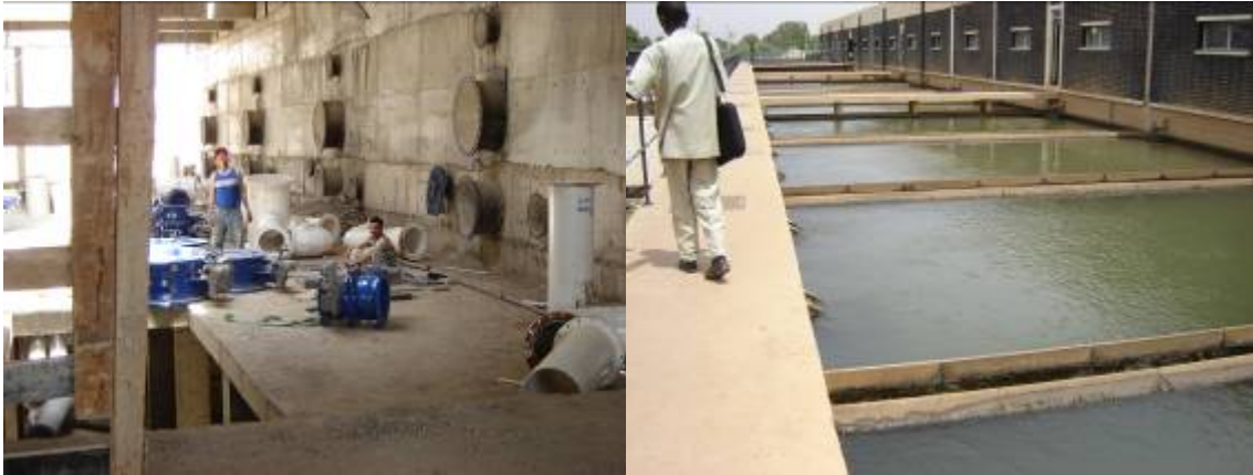
Figure 5: Gravity filters with shed (under construction) and without shed in Khartoum
