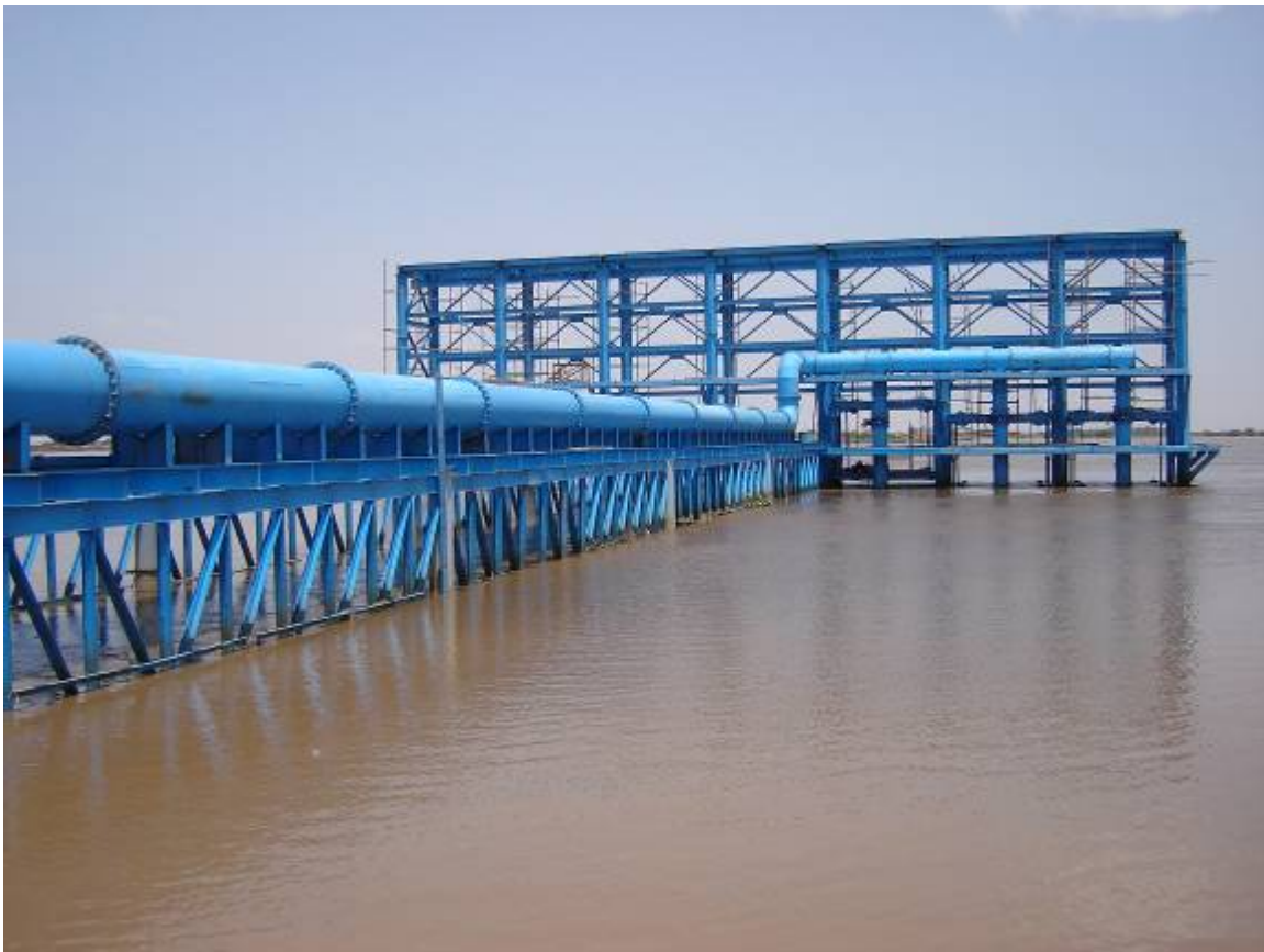
Figure 2: River intake of a treatment plant in Khartoum
