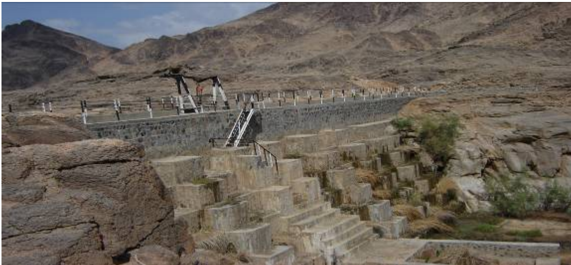
Figure 7. A masonry dam at Arbaat in Red Sea State, Sudan.
