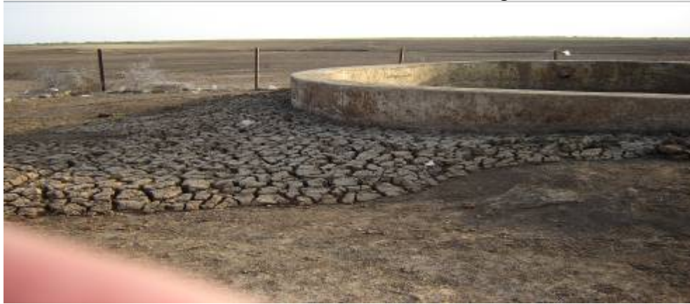
Figure 4. Sludge accumulation in the filter units and sedimentation tank of Tayba slow sand filter, Sinnar State.
