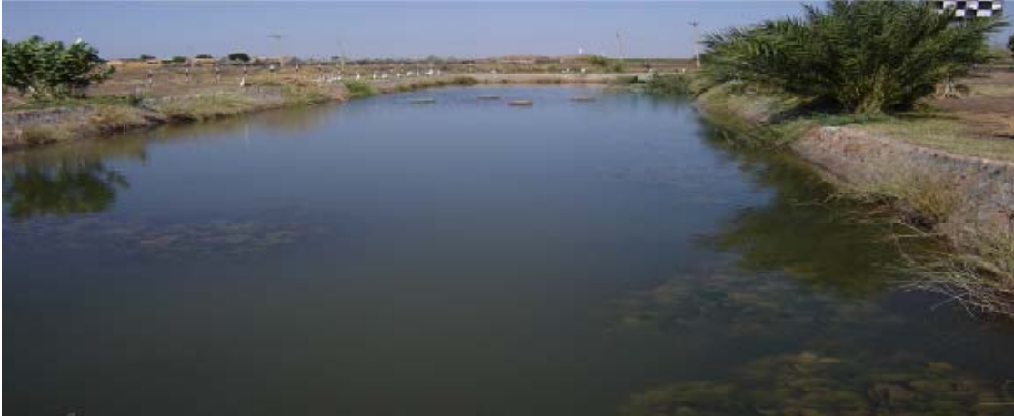
Figure 2. A pre-sedimentation basin (locally called “lagoon”) to treat water from irrigation canals in Kassala State, Sudan before the water is passed through a slow sand filter
