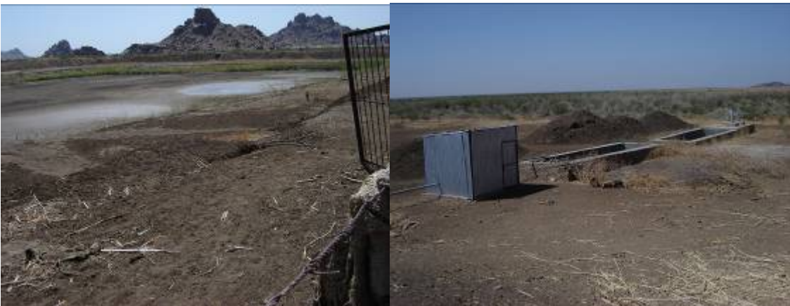
Figure 3. A hafir and its slow sand filter in Kalkalat area, Kassala State. The hafir has dried out due to the lack of rainfall
