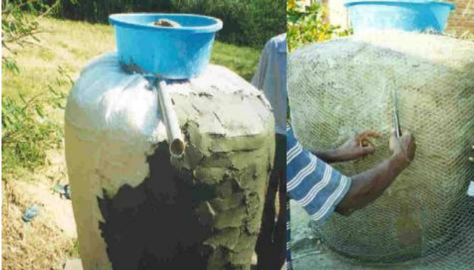
Shape formation and methods of construction of ferrocement storage reservoir (India)
