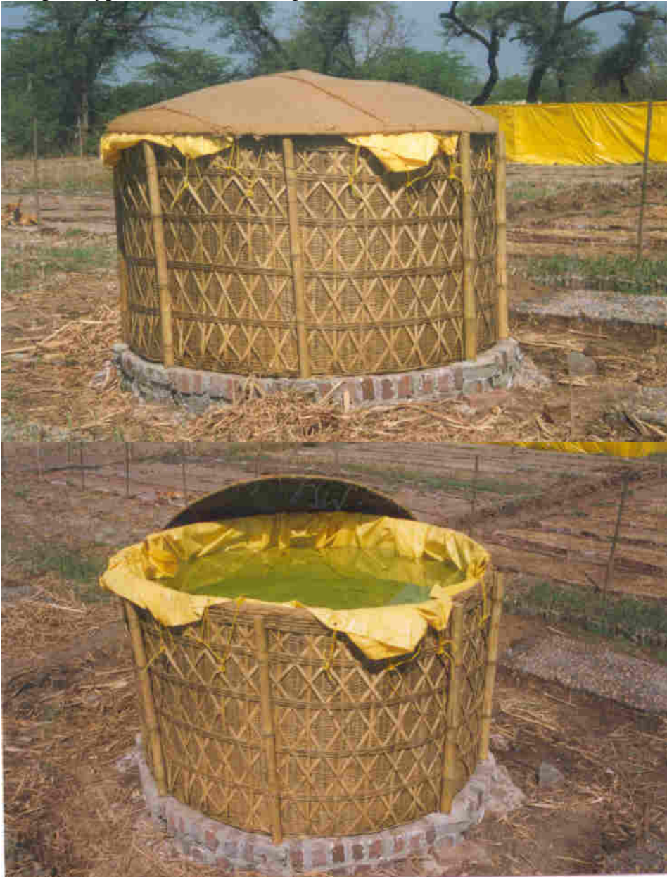
Pumpkin type ferrocement storage reservoir (Srilanka)
