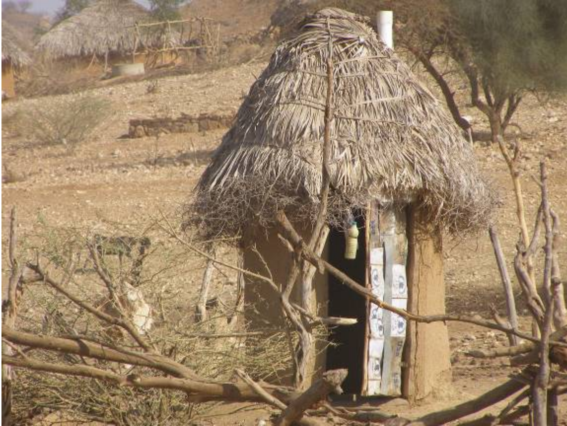
Figure 13: VIP latrine with a superstructure of mud brick wall and thatched roof
