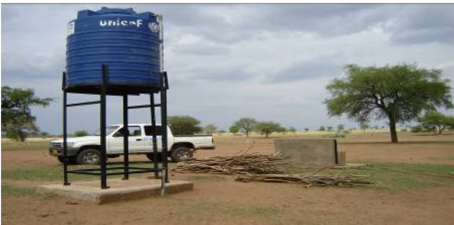
Smaller size storage facilities in South Kordofan State made from PE material
