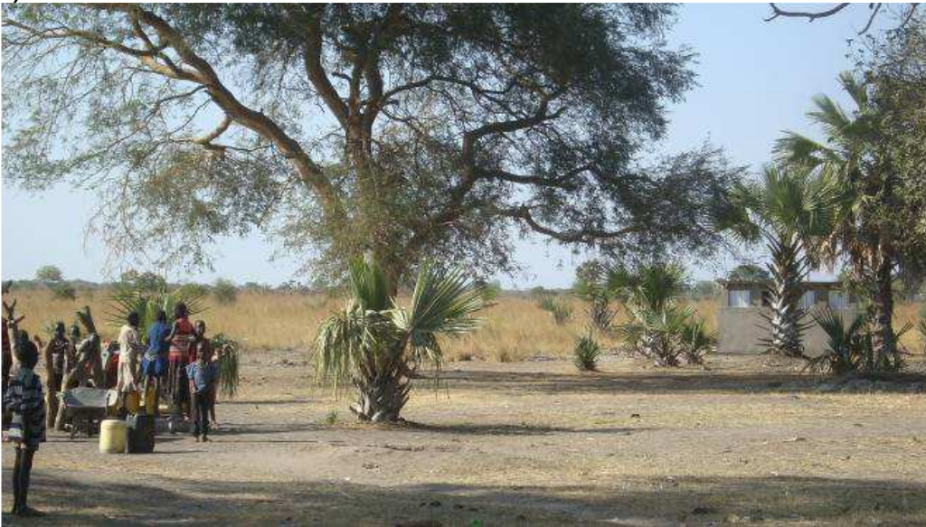
Pictures showing the finished latrines (2 male/2 female) at Payuel Primary School and water point at the foreground with 100 M between the septic and soak away. These latrines are "pour flush" and will be dependent on the water point.
