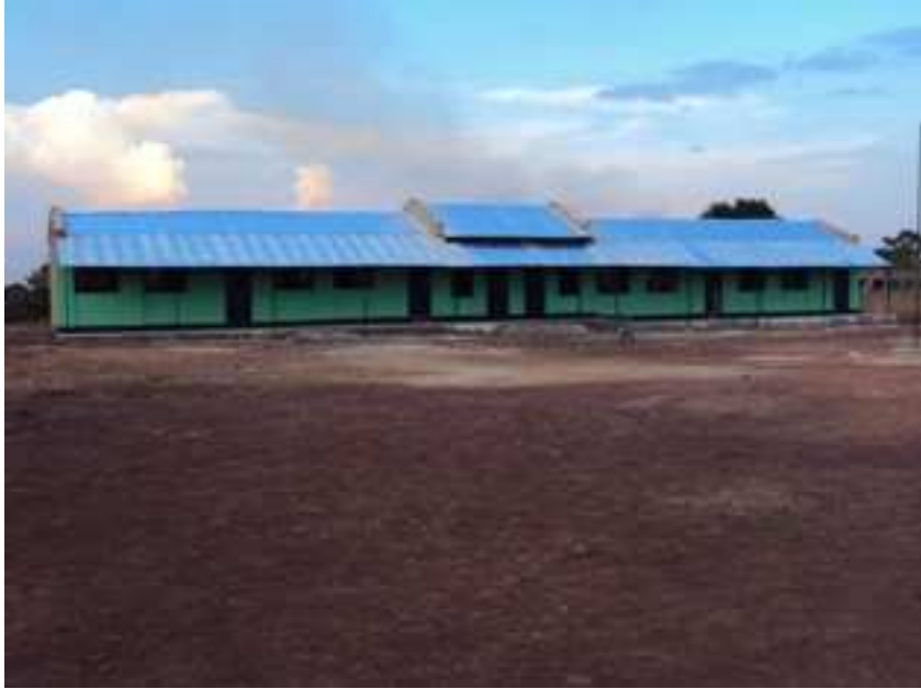
Bagari School 4 classrooms ready for use
