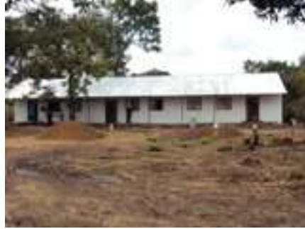
Atido Primary School 3 Class rooms
