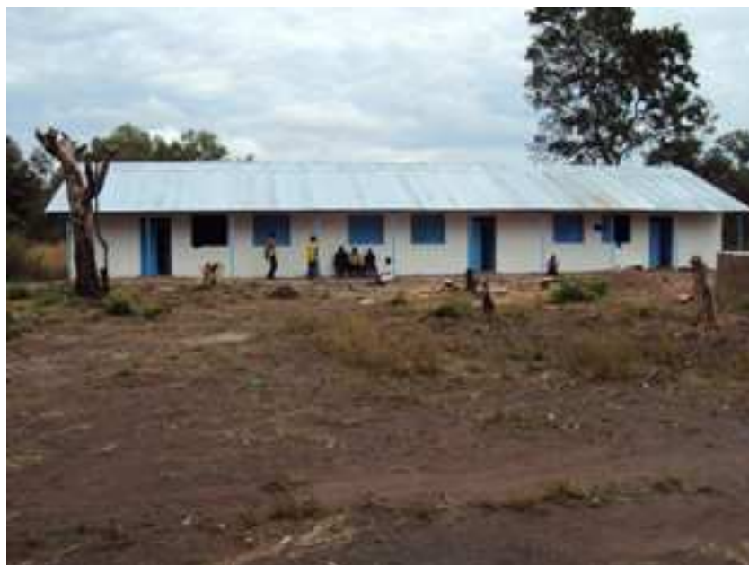
Atido Primary School 3 Class rooms
