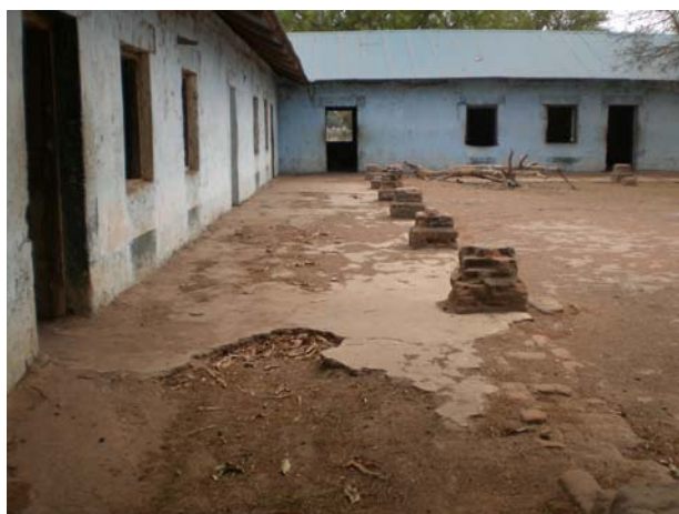
Block of 4 classrooms and one staff office before renovation
