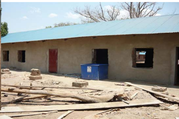
block of 4 classrooms and one staff office during renovation
