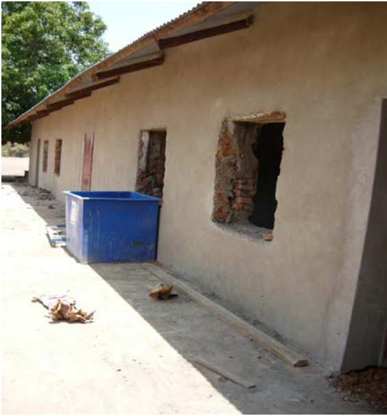
block of 4 classrooms and one staff office during renovation
